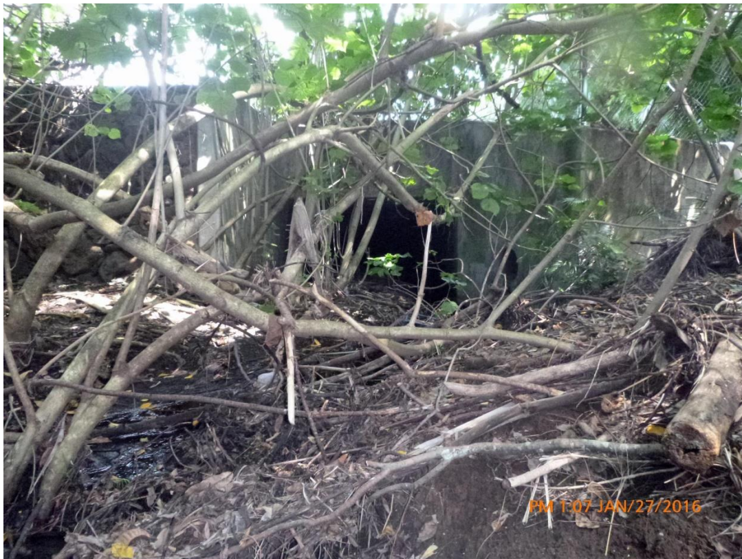
Figure 5. A box culvert discharges groundwater and storm water into Mānoa Stream in the Project area.
